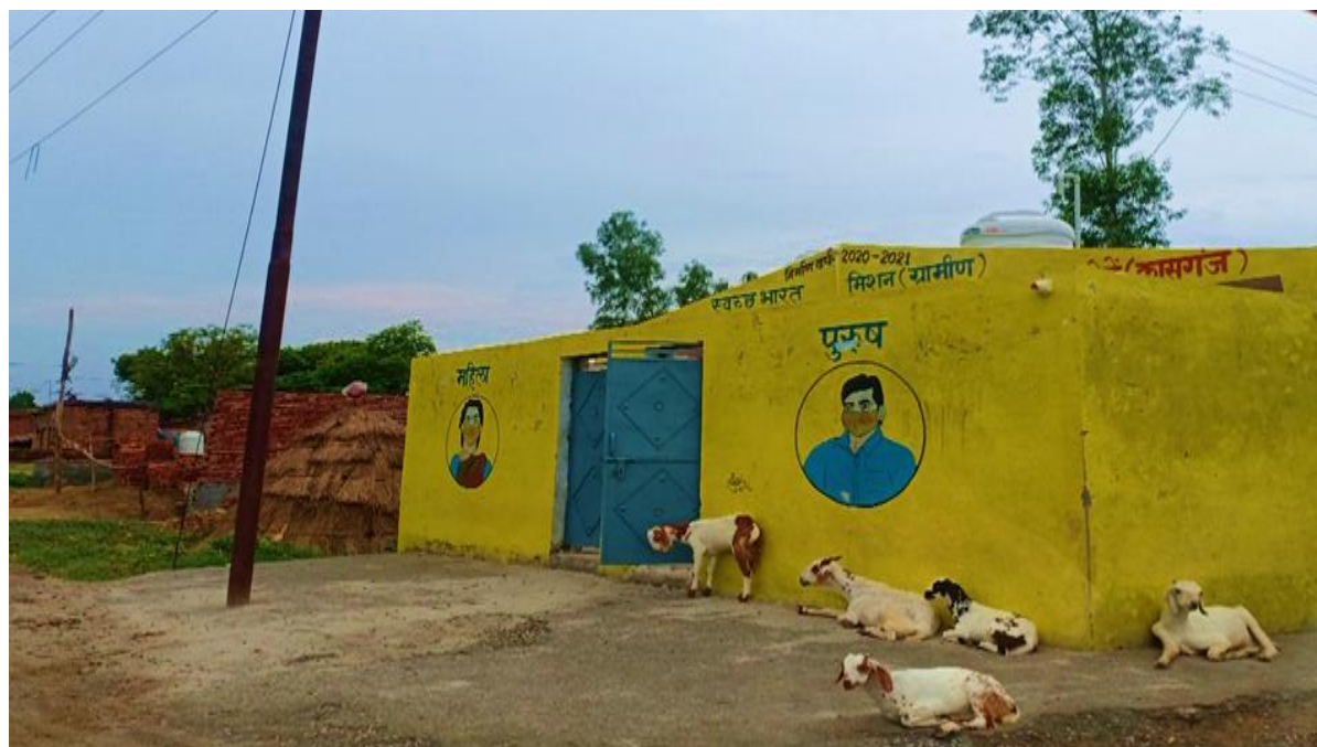
FIGURE 3.17: COMMUNITY TOILETS IN THE VILLAGES CONSTRUCTED BY STATE GOVT. VILLAGE-GOHATI
